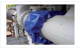
The protective cover used to mitigate the effects of possible damage to the expansion joint by stopping the leakage of medium directly into the environment.
